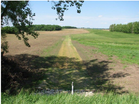
2.5 acres of Grassed Waterways installed 1 acre Critical Area Seeding installed
