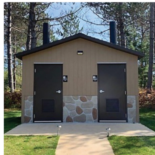
Vault Toilets for Harnischfeger & Wild Goose State Trail
