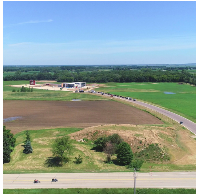
Marshland Crossing Industrial Park ft. MPTC - Horicon Regional Center
